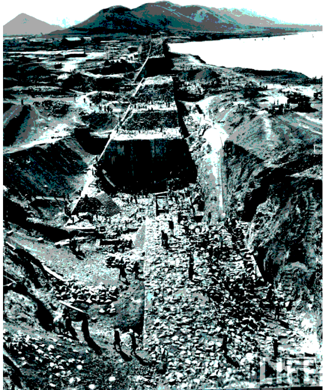
Fig 5.2 : Tungabhadra Dam Construction - 1952
